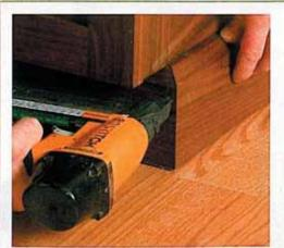
Splits are unlikely. Because they're made from such thin wire and move so fast when they're fired, 18-gauge brads are less likely to split hardwoods than hand-driven nails.
