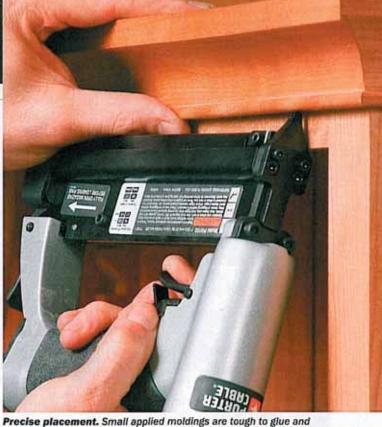
Precise placement. Small applied moldings are tough to glue and clamp, but a pin nailer with its tiny nosepiece makes it easy to hold and fasten even the smallest moldings.
